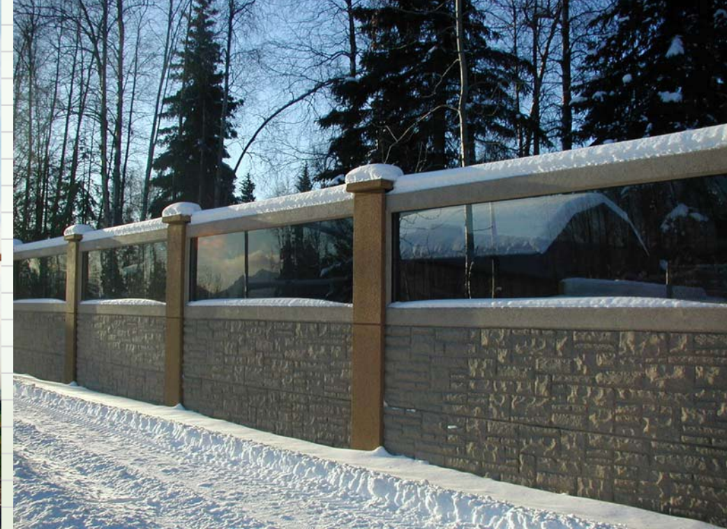
PARAGLAS SOUNDSTOP® Noise Barrier Sheet used in DURISOL® sound absorptive wall.
