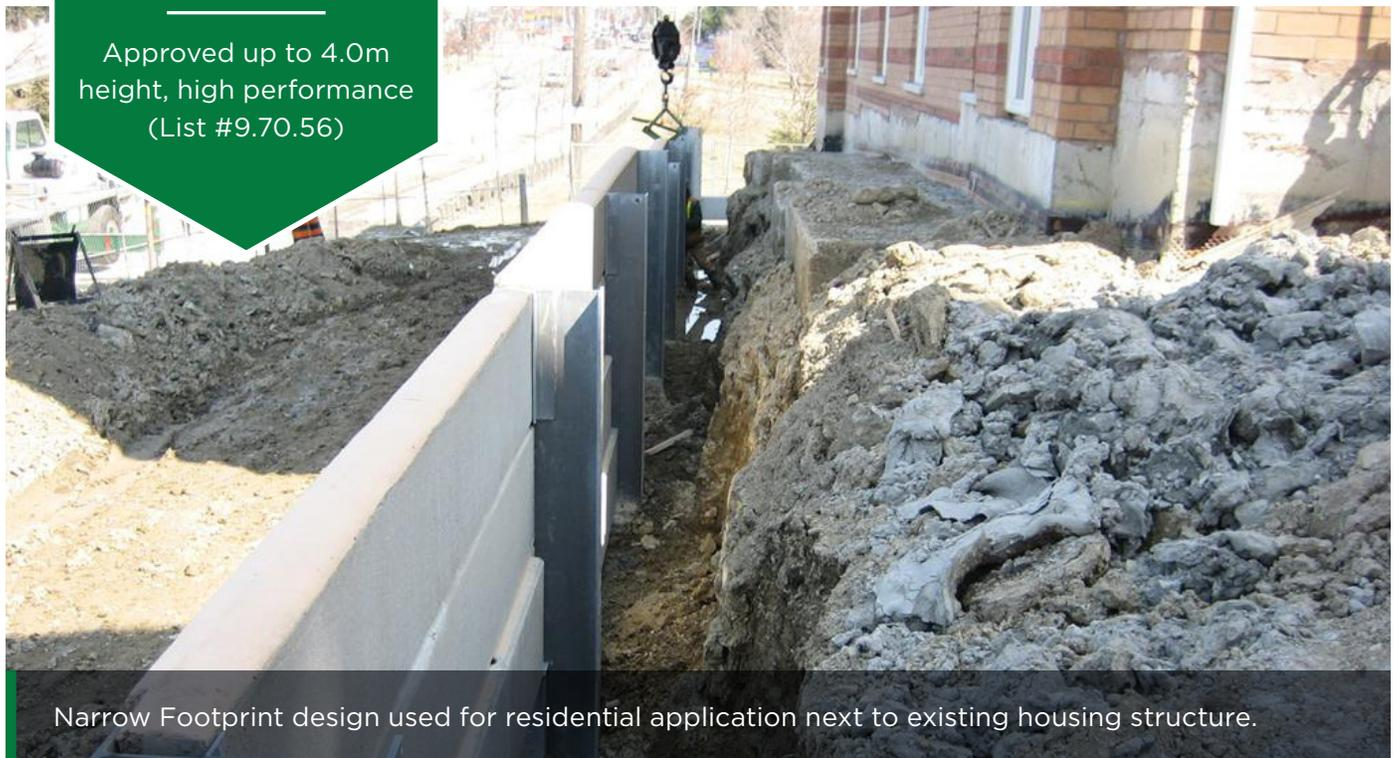
Narrow Footprint design used for residential application next to existing housing structure.
