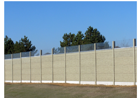
WINDSOR, ON - SOUNDSTOP NOISE BARRIER PANELS
