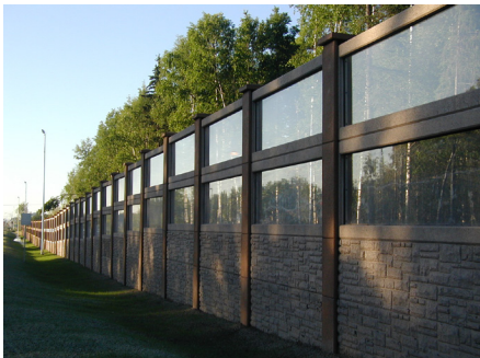
ANCHORAGE, AK - SOUNDSTOP NOISE BARRIER PANELS
