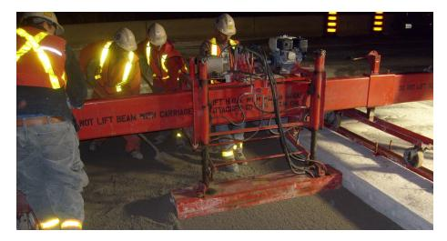
The project consisted of both intermittent and continuous repair on several areas of the QEW-HWY 427 northbound (NB) ramp and 427 (NB) Express route mainline. Normal weight precast concrete Super-Slab® panels were used for full depth replacement.
