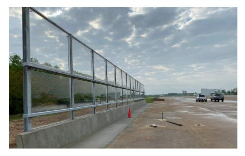
The **Durisol®-Acrylite®** Soundstop MASH TL-4 Noise Barrier System is crash-tested and contains polyamide filaments for fragment retention.
