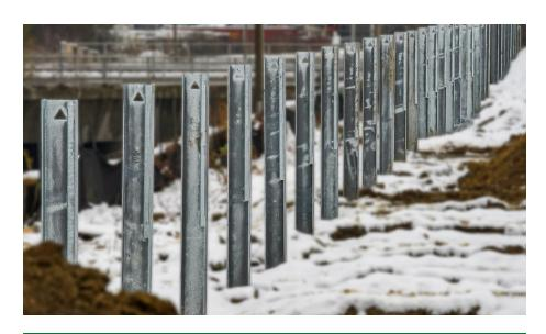
A post and panel system is more cost-effective where earth retaining heights above 1.5 metres is required.
