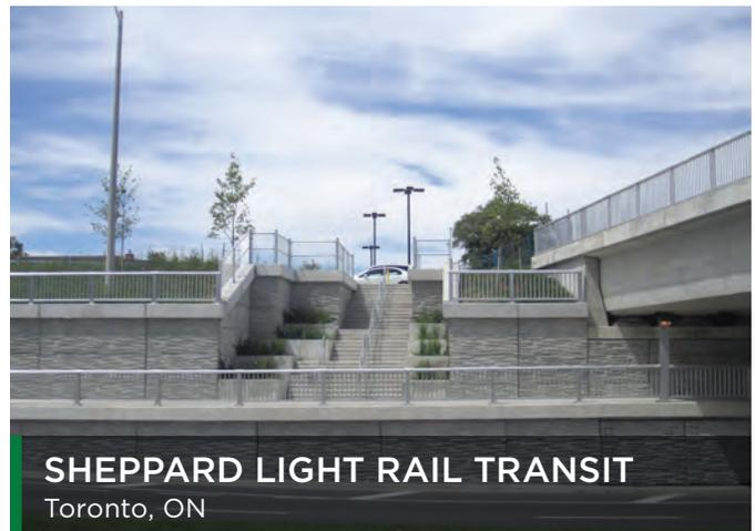
Custom patterned retaining wall panels designed to cover posts.
