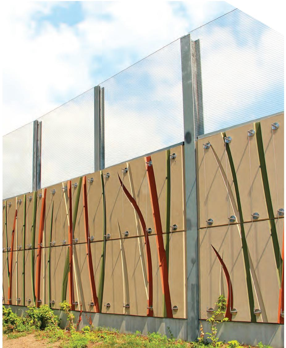
Durisol was approached by the client to engineer multiple custom wall designs in what would turn out to be the largest noise abatement project ever in North America. Over 10,000 linear metres of custom precast Durisol panels and transparent ACRYLITE® Soundstop sheets were installed along the UP Express rail corridor.
