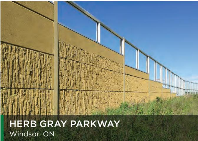
Custom Durisol panel pattern and colour integrated with ACRYLITE® Soundstop transparent sheets.
